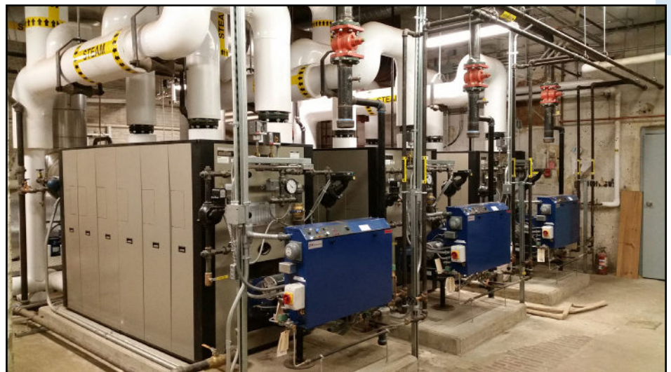
Three new Weil-McLain 88 series boilers installed in the Elm Street Elementary boiler room
