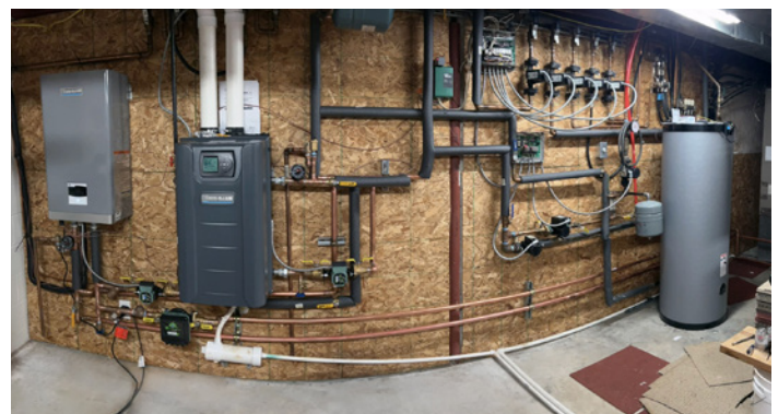
ECO HP integrated into homeowner's existing hydronic system
