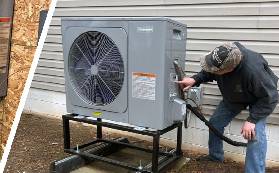
ECO HP Outdoor Unit – Air-to-Water heat pump with split design (no freeze protection required)
