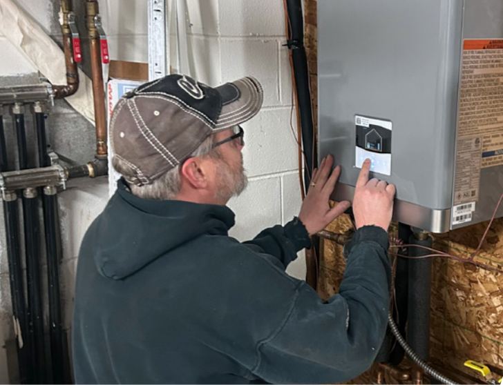
ECO HP Indoor Unit – Heat Interface Unit Integrating the heat pump into the overall system
