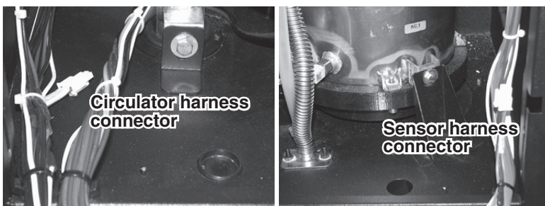
Figure 15 WM97+155 harness connector locations
