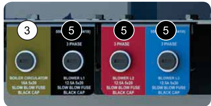
Figure 99 SVF 2500/3000 Circulator and blower fuse location
