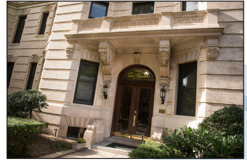
The front facade of the Mendota Apartments
