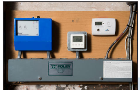
Additional controls in the Mendota boiler room
