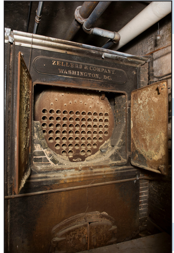
The existing steam boiler, in place for over 40 years
