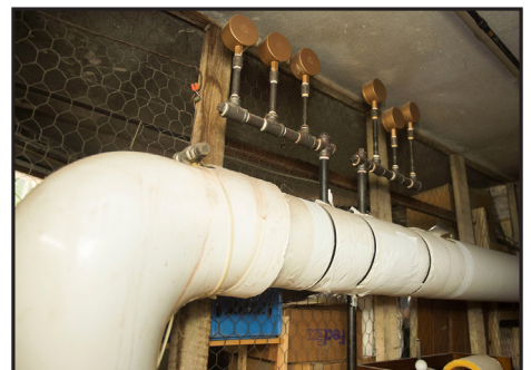
Piping and gauges in the Mendota boiler room
