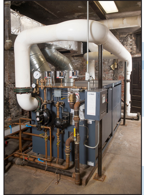
The Weil-McLain LGB-20 steam boiler in the Mendota boiler room
