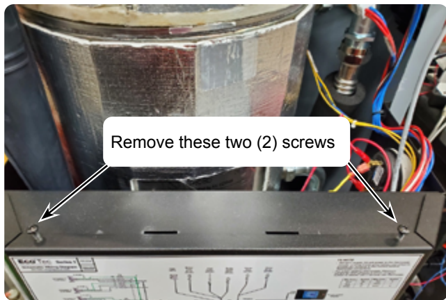
Figure 1 Removing Control Panel Cover
