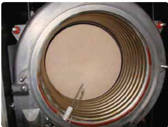
Figure 144 Inspecting and cleaning heat exchanger
