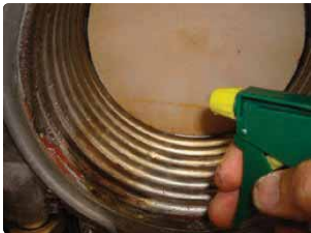
Figure 145 Cleaning the heat exchanger
