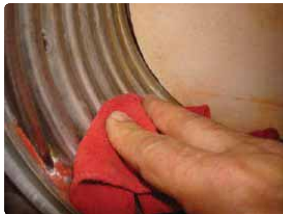
Figure 147 Cleaning the heat exchanger
