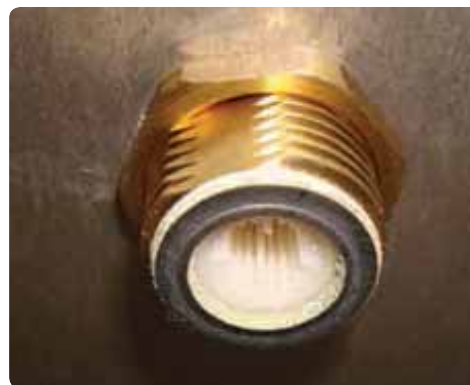
Figure 43 DHW inlet has a filter screen
