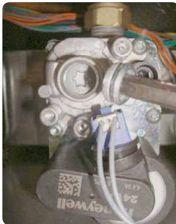
Figure 103 Remove T-40 cover cap with supplied Torx wrench for adjustment
