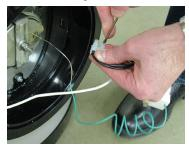
2 Insert new sensor into tank; thread new sensor wire and existing domestic water input wires through hole in faceplate.
