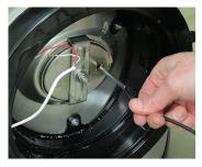
**3** Attach new sensor wire and domestic water input wire to new control.
