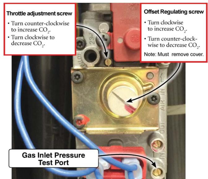
Do NOT attempt to bottom out the offset regulating screw as was done for the throttle adjustment.
