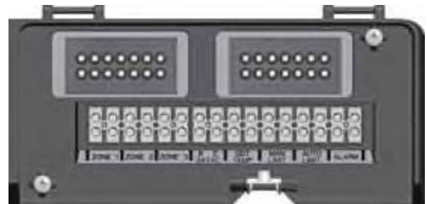
Low voltage wiring terminals
