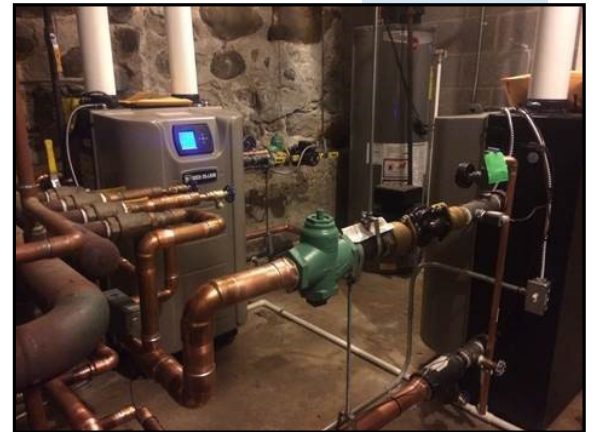
The two Evergreen units installed in the boiler room provide energy efficient heating for the church
