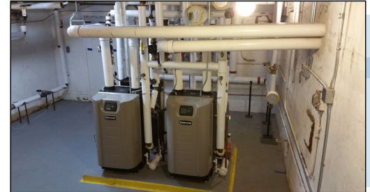
Three new Evergreen 399 boilers in the Weyhill Guest House boiler room
