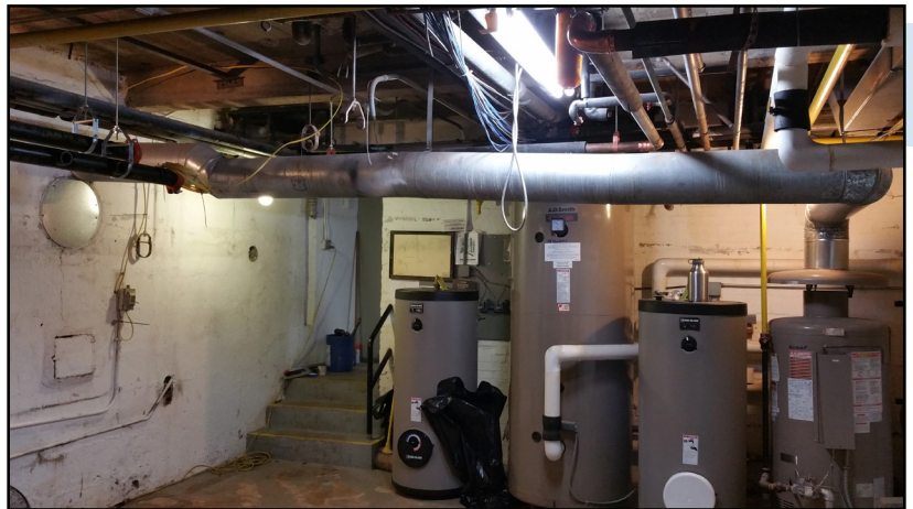
Two new Aqua Plus water heaters in the Weyhill Guest House boiler room
