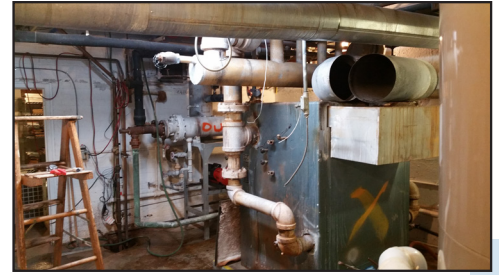
The existing steam boiler in the Weyhill Guest House boiler room, prior to installation of the new equipment
