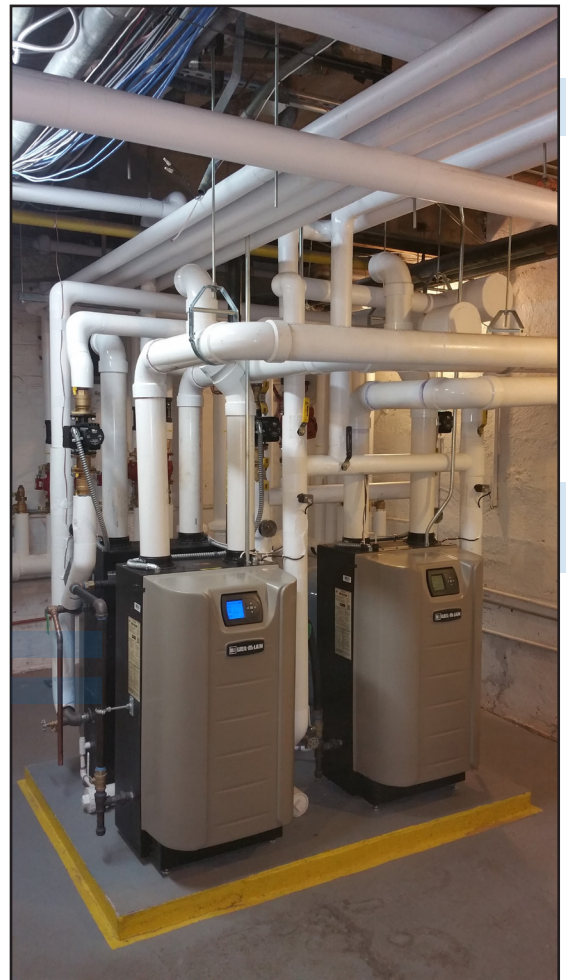
Three new Evergreen 399 boilers in the Weyhill Guest House boiler room
