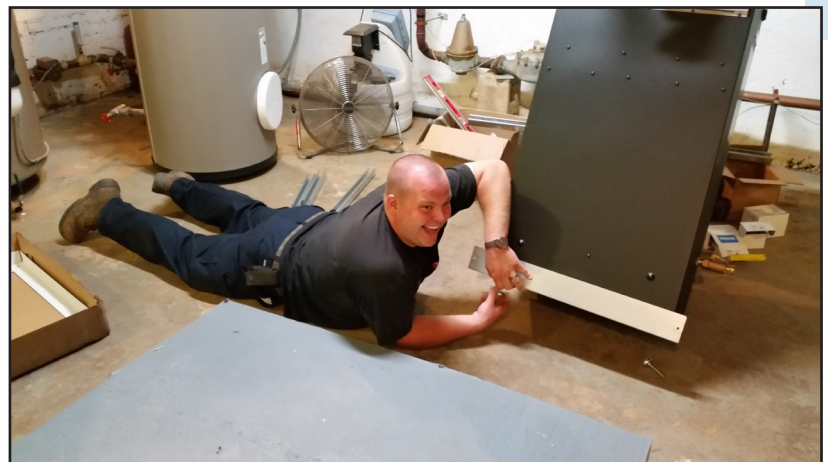
Dakota Brown from eastern Pennsylvania-based contractor Dual Temp installing the new equipment
