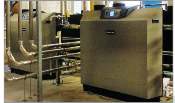
2 of the 4 Ultra™ 750 boilers
