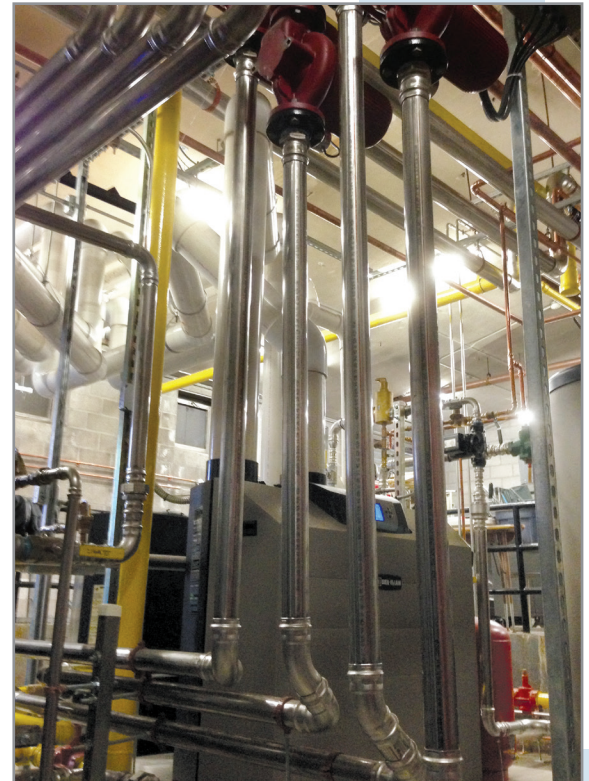
Ultra™ 750 boiler and new stainless steel piping
