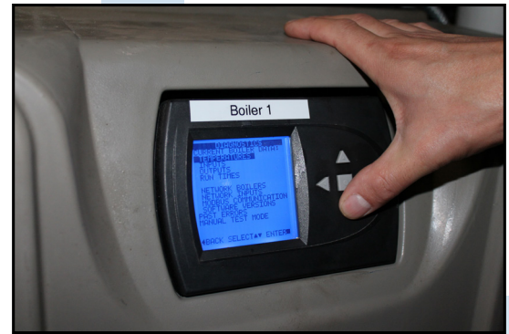
A close-up of the easy to navigate Evergreen boiler controls and interface
