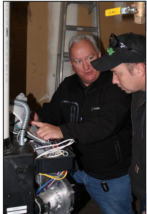
Weil-McLain Commercial Specialist Mike Gambill assists with maintenance training on the new Evergreen units
