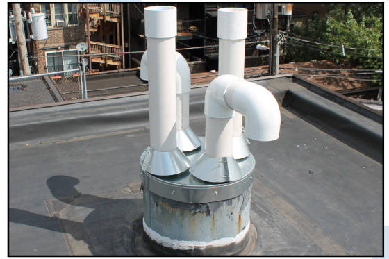
The intake and exhaust pipes vented through the roof of the Presence Health Medical Facility
