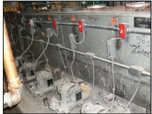
The existing Multi-Temp boilers which were originally installed prior to this project
