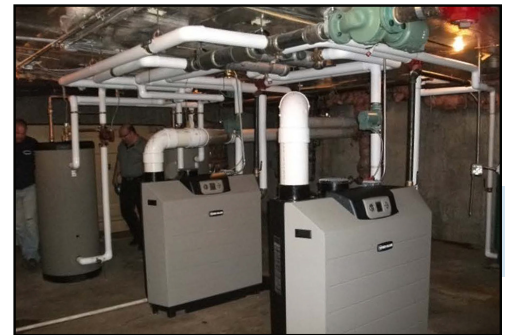
New SlimFit 750 boilers and Aqua PLUS water heater installed in one of the boiler rooms
